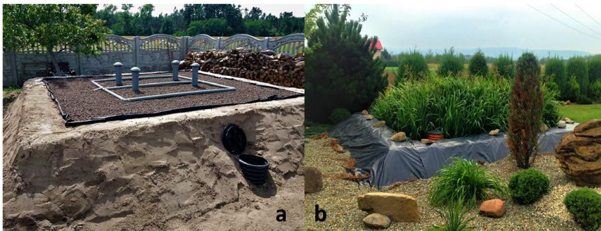
Figure 3 LECA-based Vertical Flow Constructed Wetland before (a) and after (b) commissioning. LECA has become one of the most commonly applied substrates for small scale, domestic CWs systems, which account for roughly 3000 units in Poland alone ( personal communication ). (Photo. F. Bydalek/ Ecoverde Engineering Office, Poland).
